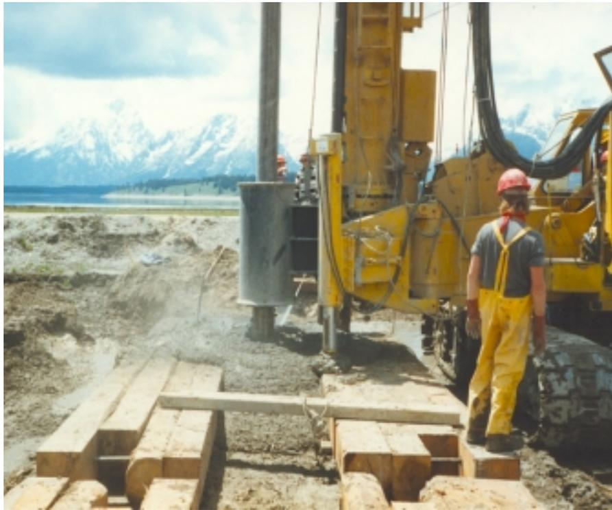
Figure 5. Soil Mixing in Progress
