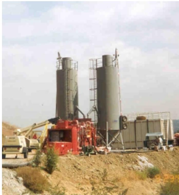
Figure 2. Central Grout Mix Plant
