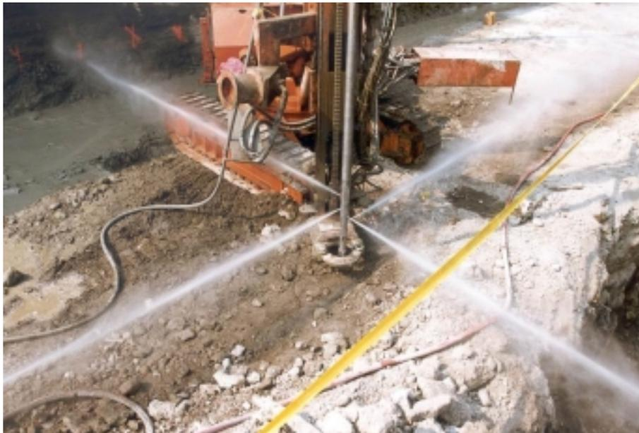
Figure 2. Jet Grout Monitor
