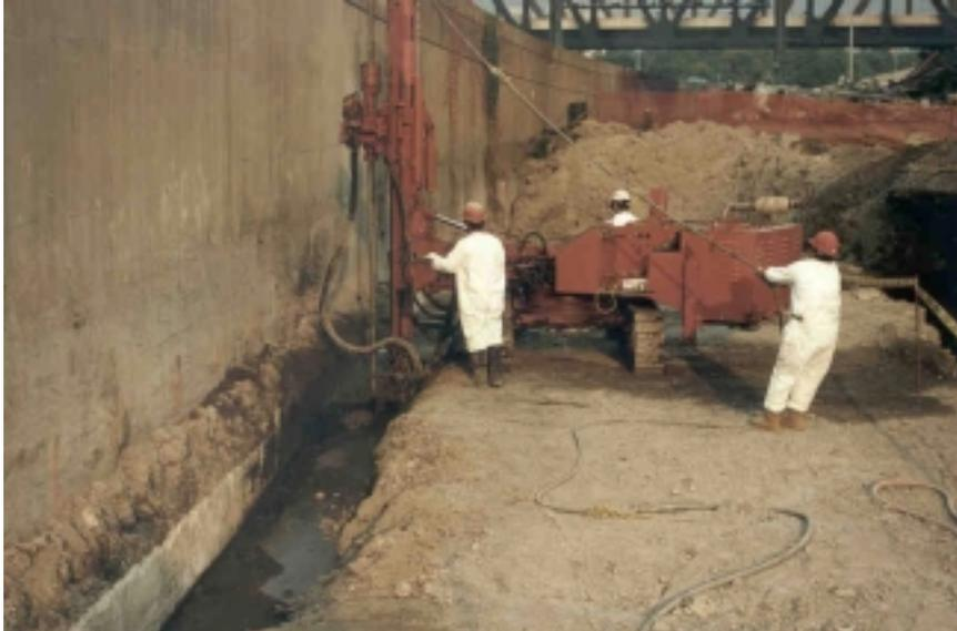
Figure 5. Jet Grouting in Progress
