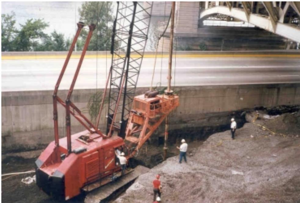
Figure 4. SSM Rig in Operation
