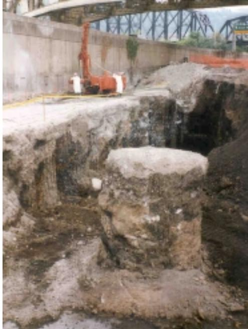
Figure 6. Trial SSM Column with Completed Wall to Left
