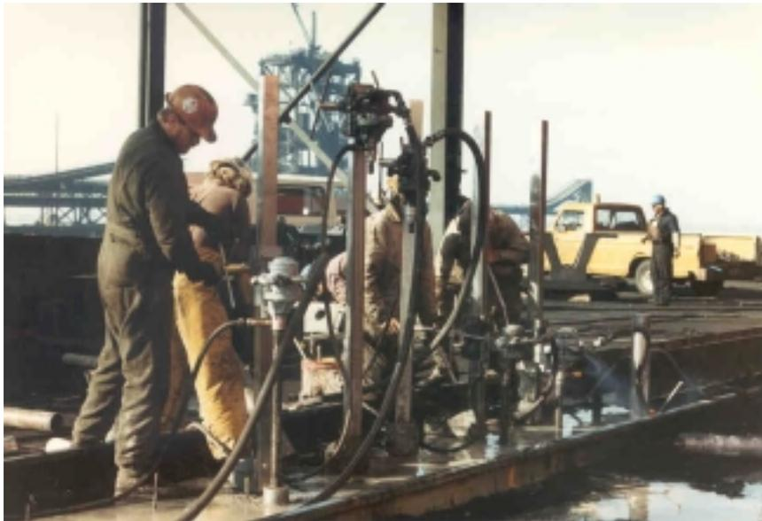
**Figure 6. Coring of Access Holes Through Pier**
