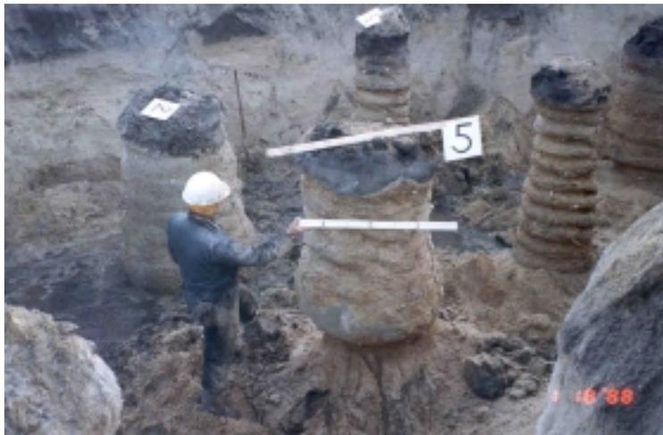
**Figure 4. Portion of Test Program Soilcrete Columns**
