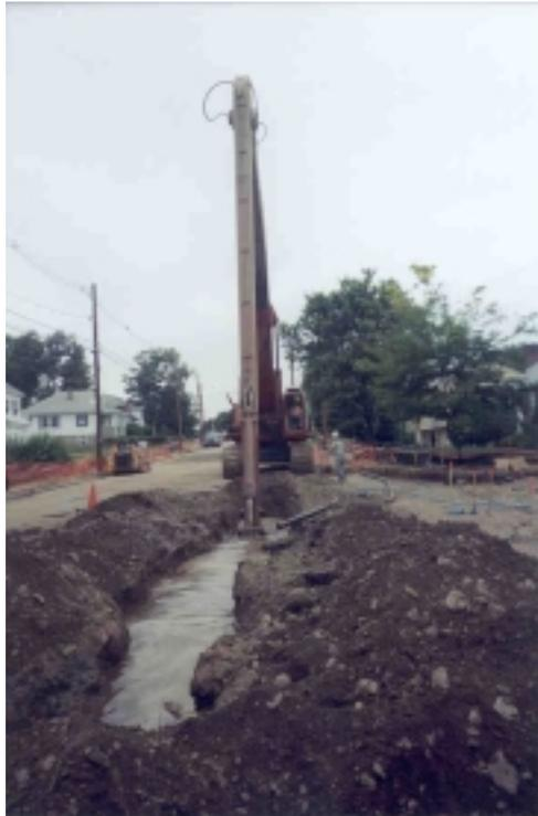
Figure 7. View of Slurry Trench Installation
