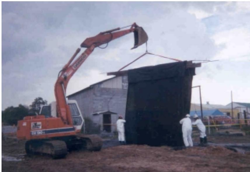
Figure 3. Installation of Geomembrane Panel
