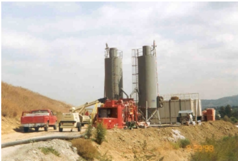
Figure 3. DSM Mix Plant
