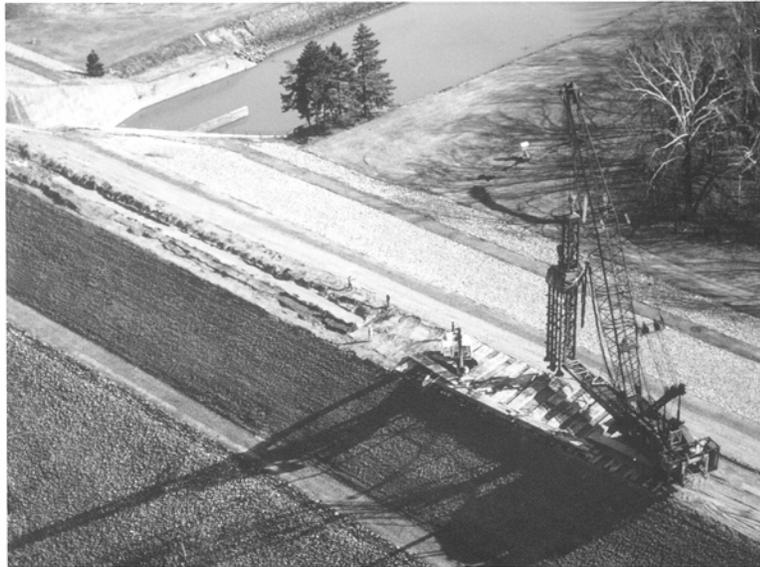
**Figure 4. DSM Unit in Operation**
