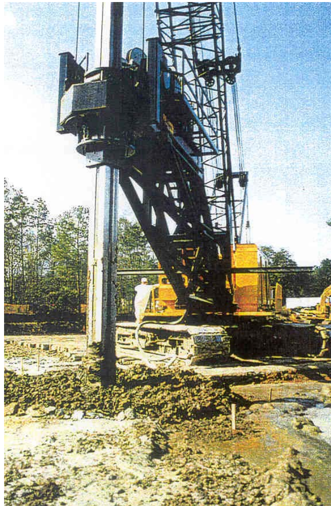
FIGURE 3 – SINGLE AUGER CAISSON-TYPE DRILL RIG
