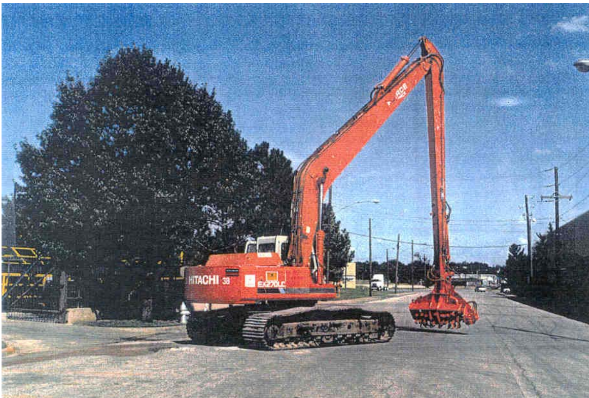
FIGURE 2 – EXCAVATOR-MOUNTED ROTARY MIXER (Photo courtesy of ITEX Environmental Services, Inc.)
