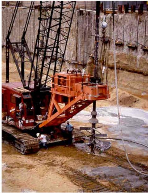
**Figure 1. Shallow Soil Mixing Equipment**
